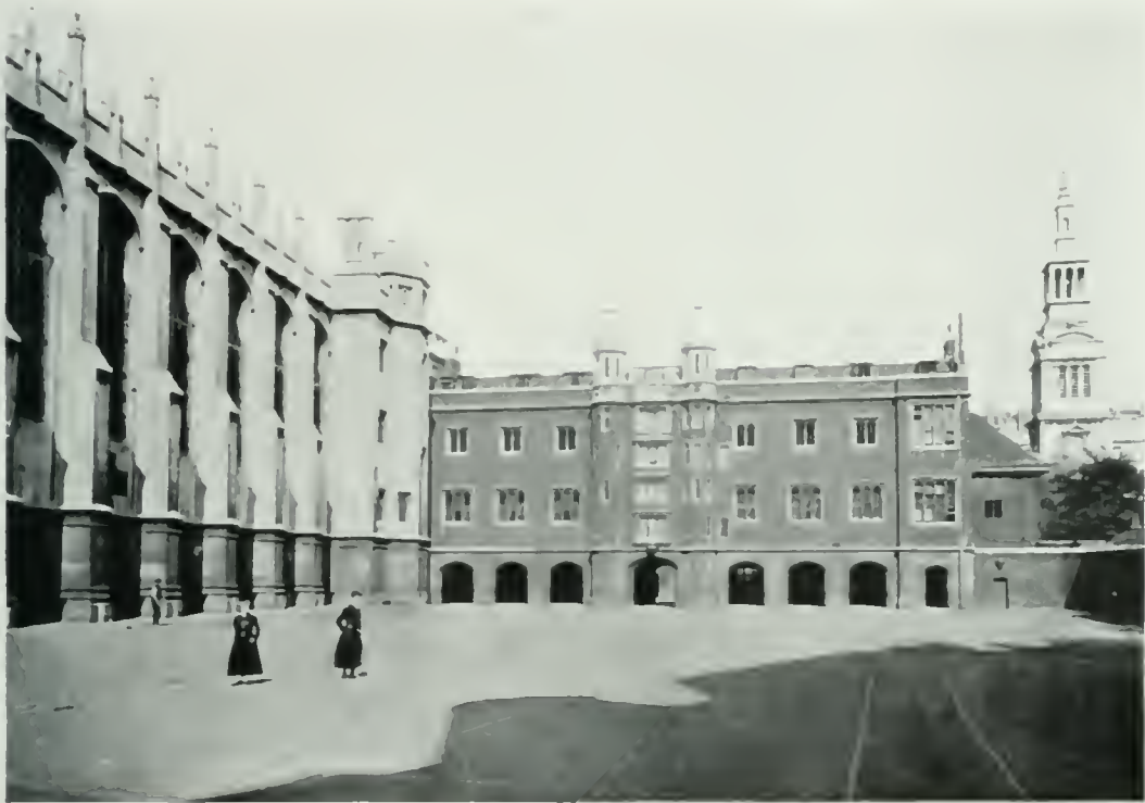
CHRIST'S HOSPITAL SHORTLY BEFORE ITS DEMOLITION, WITH THE TOWER OF CHRIST CHURCH AFTER THE REMOVAL OF THE PINNACLES.
